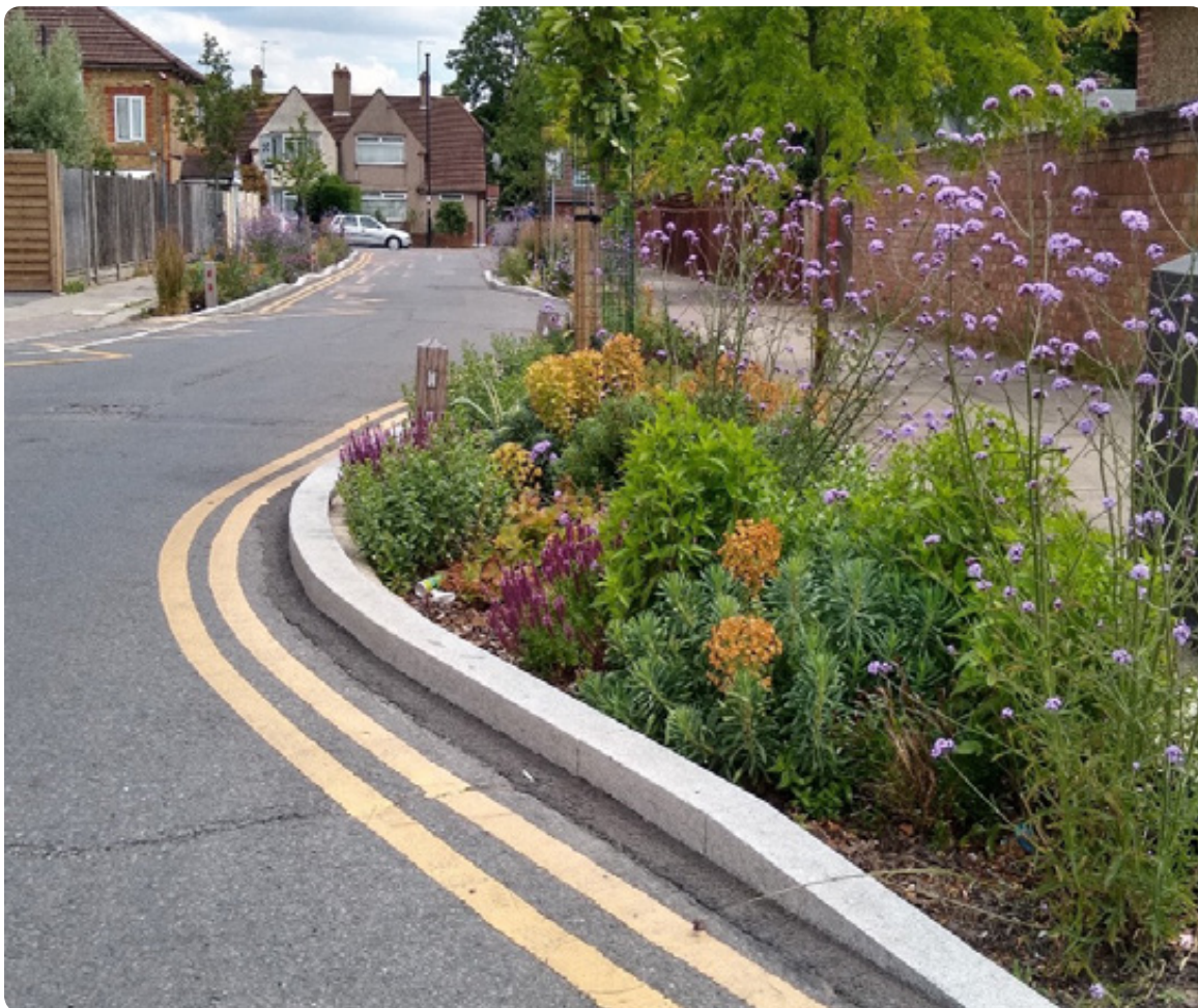
Figure 37: Rain gardens at Haselbury Road
