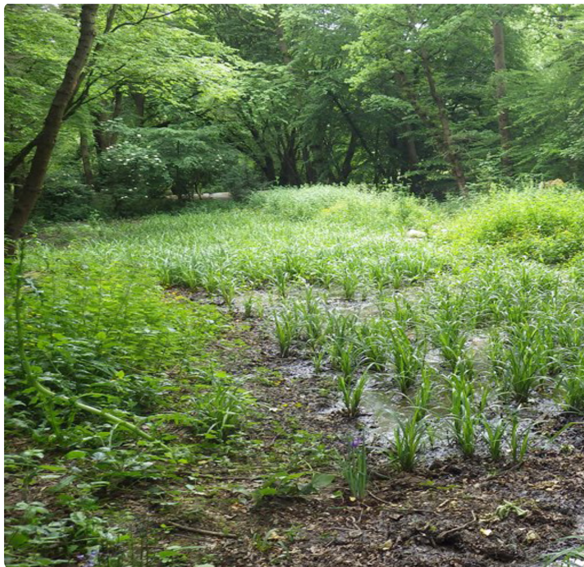
Figure 28: Sustainable urban drainage at Grovelands Park
